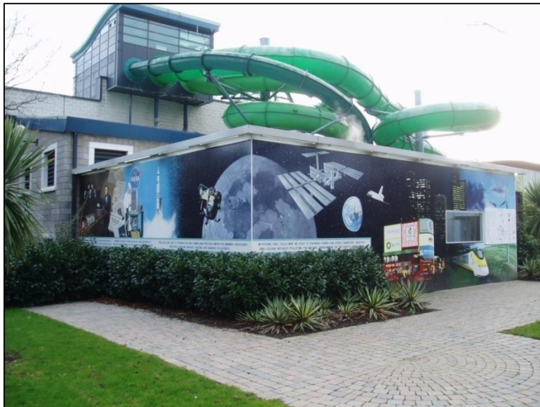
Basen w Park Fuel Cell CHP
