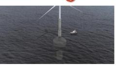
**TELWIND** integrates floating substructure and a selferecting telescopic tower. It allows for a full onshore preassembly of the overall system, ensuring reduction of offshore works and auxiliary means.
